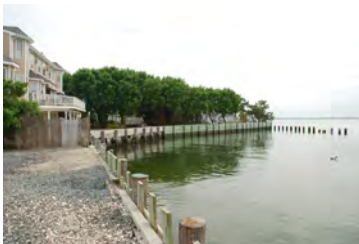
Figure 38 Both public and private investments are needed to keep Oxford's maritime infrastructure in good working order
