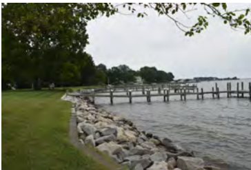
Figure 29 Hardened shorelines along the more exposed Tred Avon River waterfront
