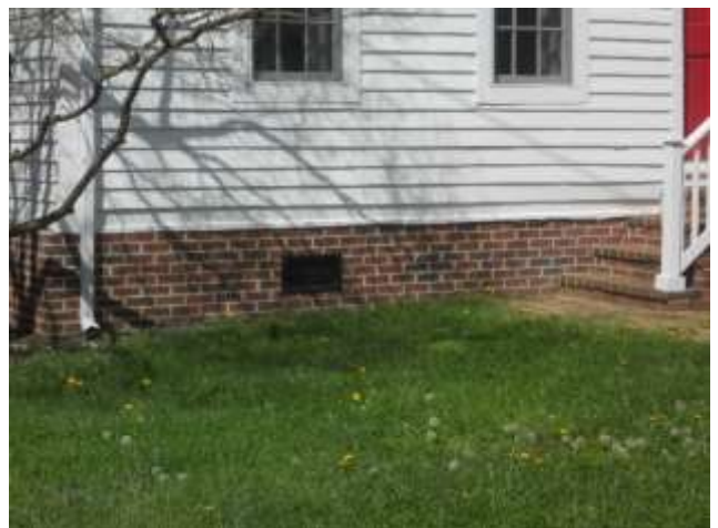
Typical Brick Foundation with Flood Venting
