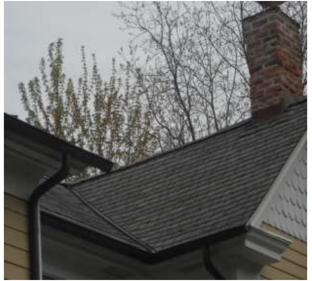
Asphalt Shingle Roofing with Metal Valleys
