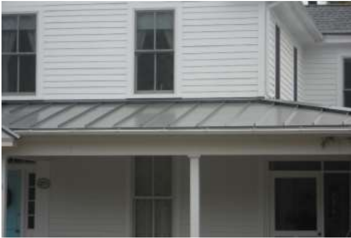
Standing Seam Metal Roofing
