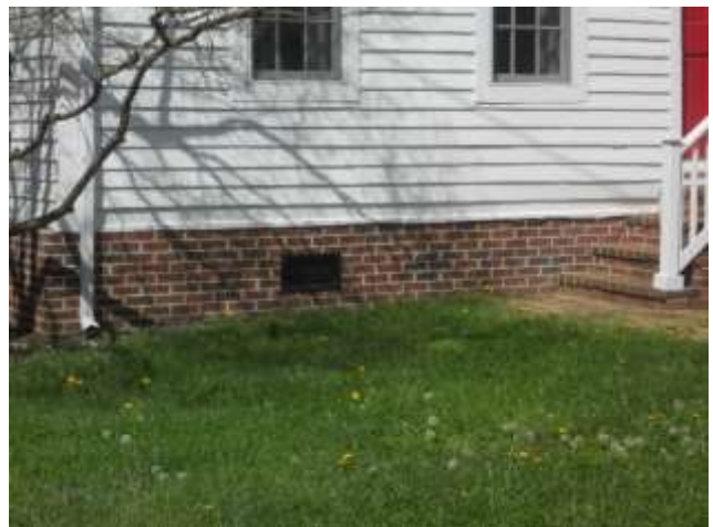
Typical Brick Foundation with Flood Venting
