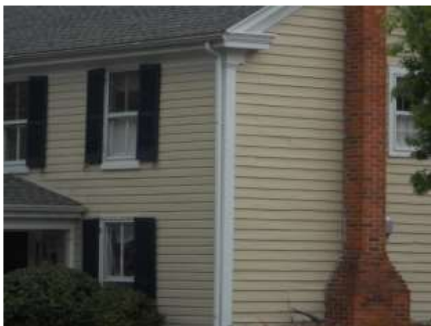
Clapboard Siding with Corner Board
