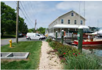
Figure 15 Tide gate (left) installed near Hinckley's Yacht Services on Bank Street
