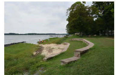
Figure 19 Living shoreline installed along the Tred Avon River at the Oxford Town Park
