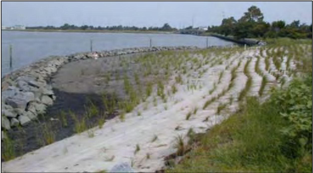
Fig. V.A.6.1. Photograph of rock sill and marsh transplanting two years post-construction in North Carolina (Source: Currin, Chapel, & Deaton, 2010).
