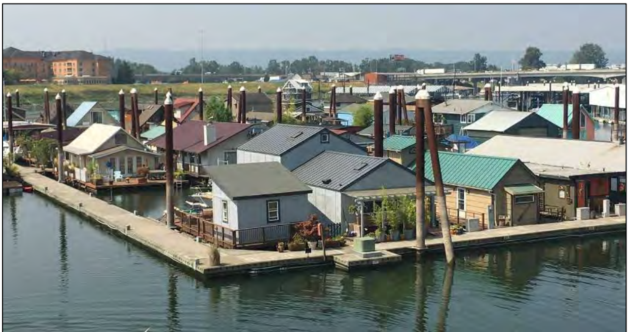
Figure V.C.4. Floating homes located in the Portland, Oregon (Source: https://pdxtoday.6amcity.com/life-floating-home-portland-oregon )
