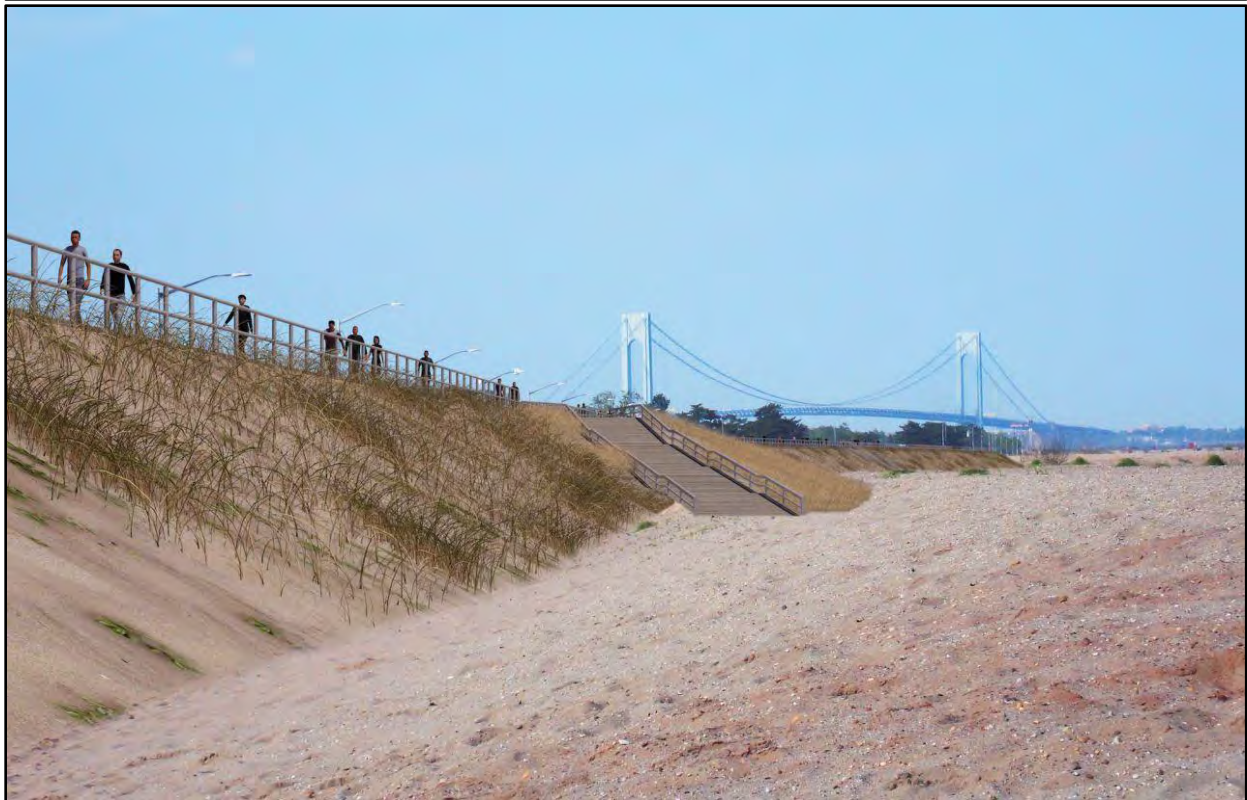
Fig. V.A.4.2. Renderings of a proposed engineered dune system/seawall able to withstand the 300-YR flood event in Staten Island, New York
