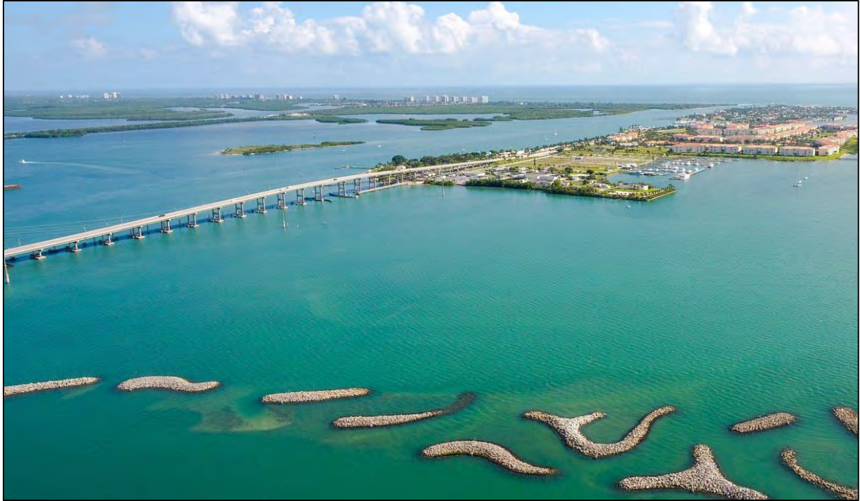
Fig. V.A.9.1. Photograph of modern curved breakwater islands and tee-shaped groin design in Fort Pierce Marina, Florida. The “hard” engineering is offset slightly by 21 acres of new habitat for oysters, mangroves, dune grass, and seagrass, as well as nesting grounds for birds (Source : https://www.cnn.com/style/article/staten-island-seawall-climate-crisis-design/index.html )
