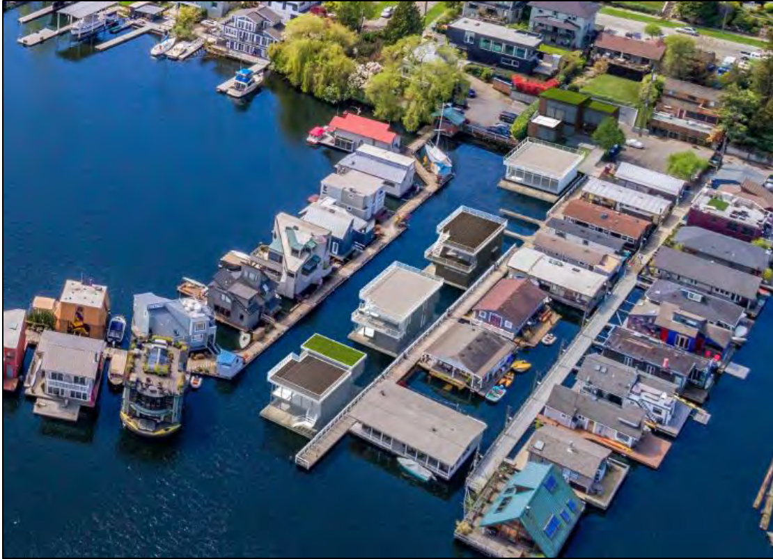
Figure V.C.5. Floating homes located in Seattle, Washington
