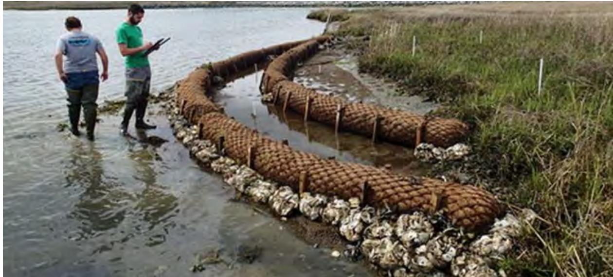
Fig. V.A.5.1. Photograph of a living shoreline project in Delaware with fiber logs, installed to protect the marsh edge
