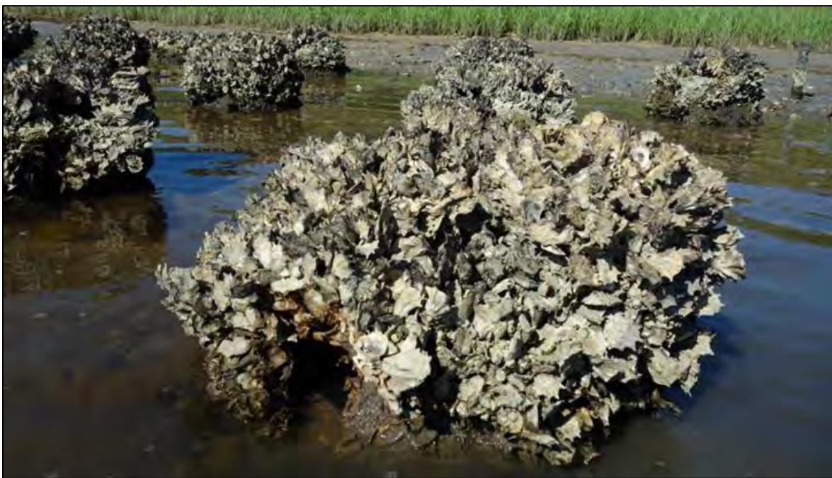
Fig. V.A.9.2. Photograph depicting a living breakwater system constructed with oyster shells (Source: https://reefinnovations.com/services/ecosystem-restoration/living-shoreline-reef-balls-are-being-used-across-the-coast )
