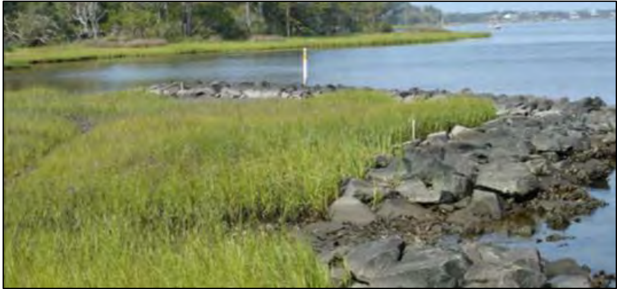
Fig. V.A.7.1. Photograph depicting toe revetment in North Carolina (Source: Currin, Chapel, & Deaton, 2010).
