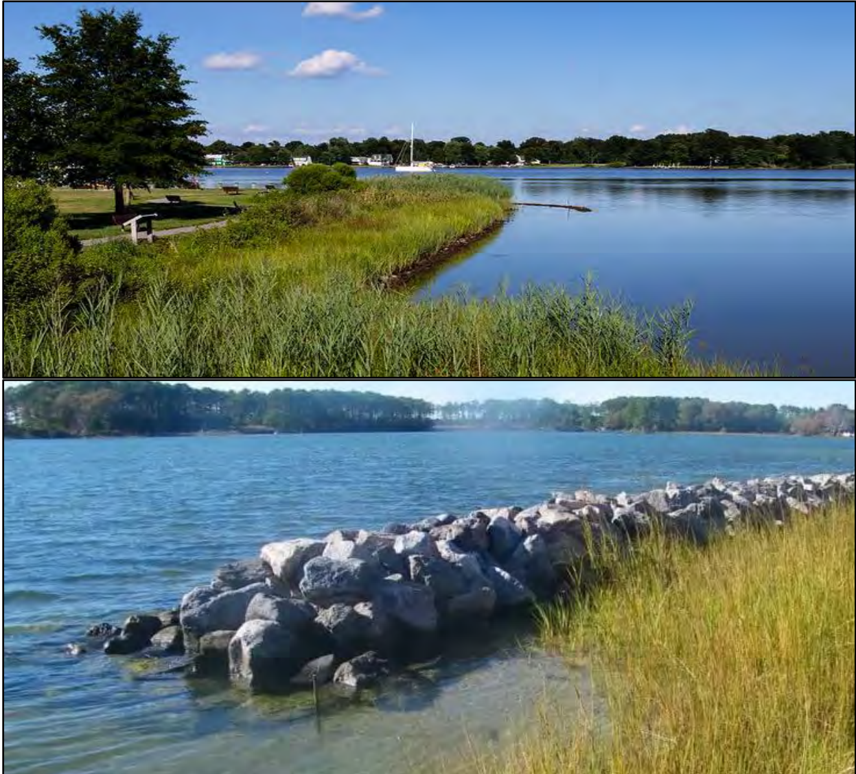
Fig. V.A.3. (a) An example of “soft” shorelines and (b) an example of hybrid shorelines (Source: (a) https://chesapeakebaymagazine.com/md-lawmakers-push-bill-to-strengthen-living-shorelines/ ; (b) https://chesapeakebaymagazine.com/state-guidance-va-waterfront-homeowners-must-use-living-shorelines-when-ever-possible/ )
