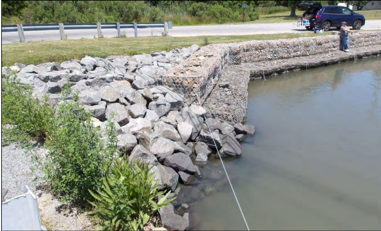
Fig. V.A.11.4. Photograph depicting a gabion sill stabilized shoreline (Photo credit: Brent Jett).
