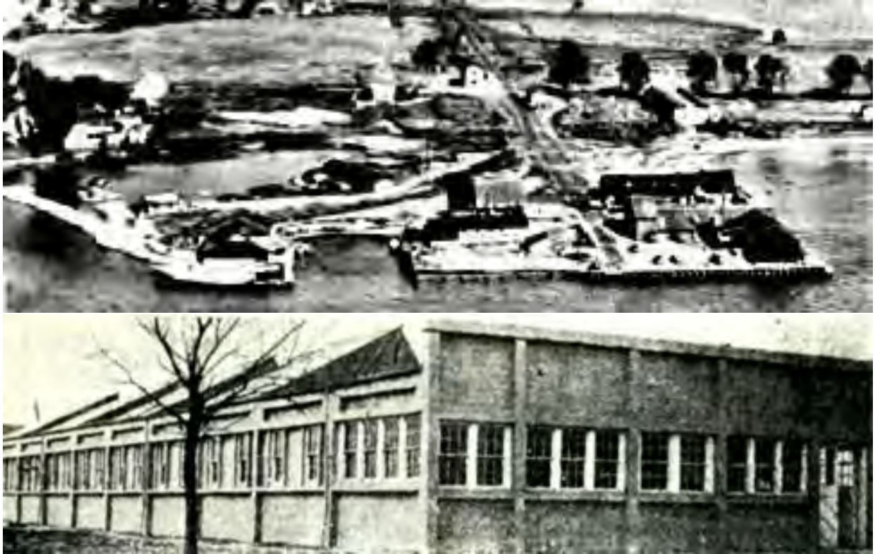
Fig. I.F.1. Aerial & Profile of Kuehner Engine Manufacturing Plant (Source: THE KUHNER ENGINE COMPANY - Gas Engine Magazine )
