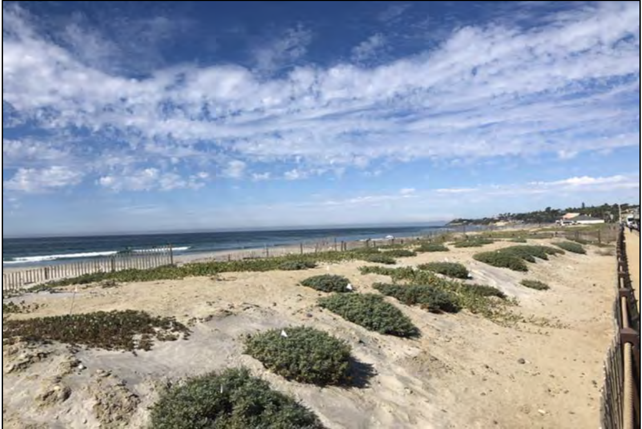
Fig. V.A.4.1. An engineered dune system in Encinitas, California designed to protect Pacific Coast Highway and enhance beach habitat.
