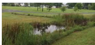
A bioswale, located in Causeway Park, filled with stormwater following a rain event. (Source NOAA)
