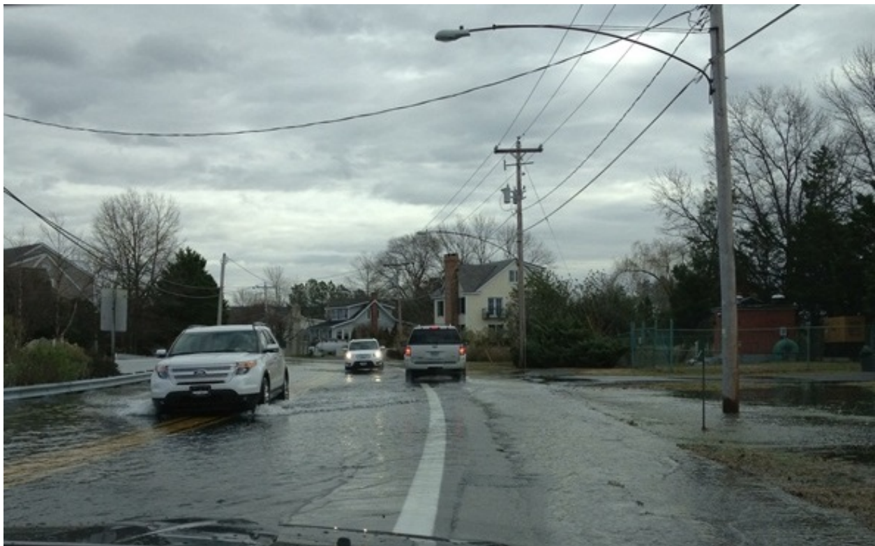
Flooded conditions along The Causeway (Photo provided by Cheryl Lewis)
