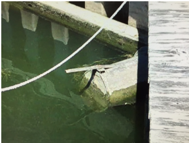
Tide Gate at West Pier Street (Photo taken by GMB)
