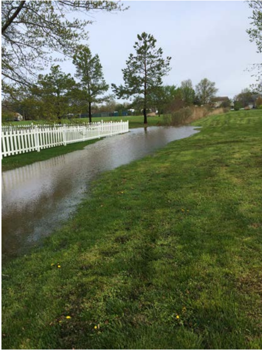
Flooded conditions between Causeway Park and Pier St (Photo provided by Cheryl Lewis)
