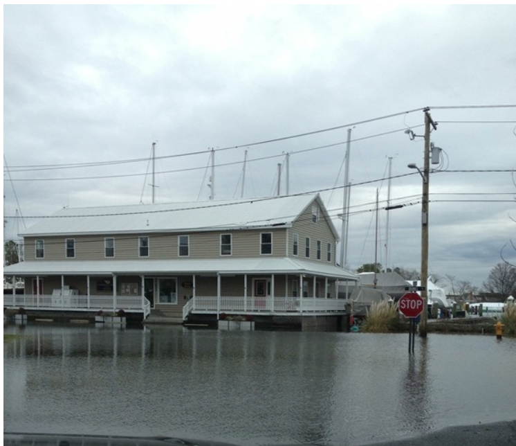
Flooded conditions at intersection of Banks and Wilson Streets (Photo provided by Cheryl Lewis)
