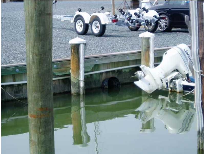
Mill Street Outfall (Photo by GMB)
