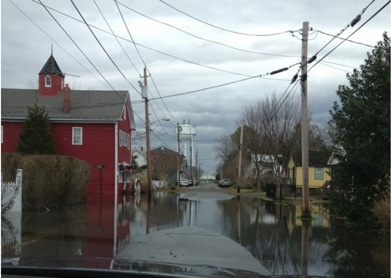
Flooded conditions at intersection of Tilghman and Stewart Streets (Photo provided by Cheryl Lewis)
