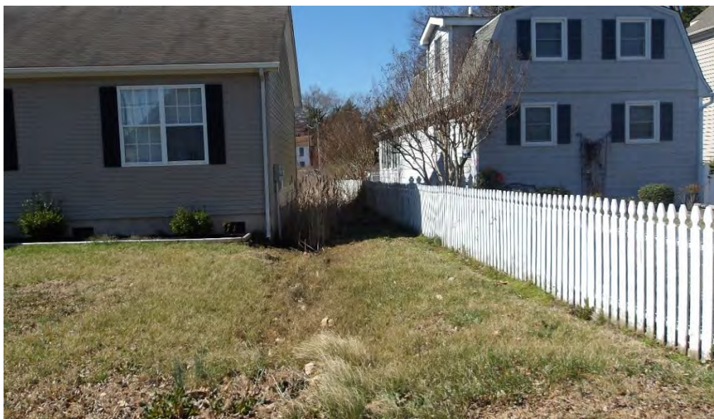
Ditch adjacent to a house in Study Area 2.
